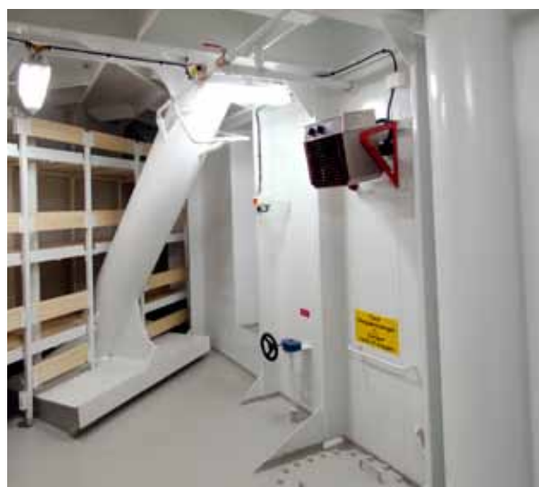
Vibrations onboard ships and offshore platforms can cause electronic equipment to malfunction. Elektra V fan heater has been designed to overcome these stresses.
