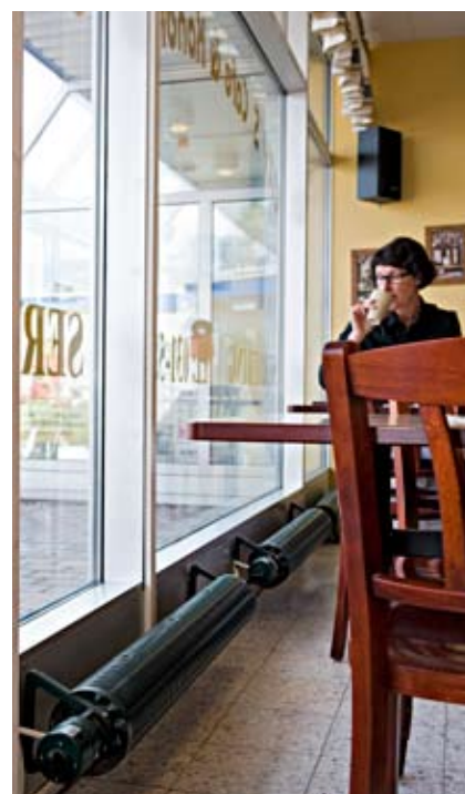
The ribbed pipe radiator's design and mounting brackets make them easy to install, for example, below a window.
